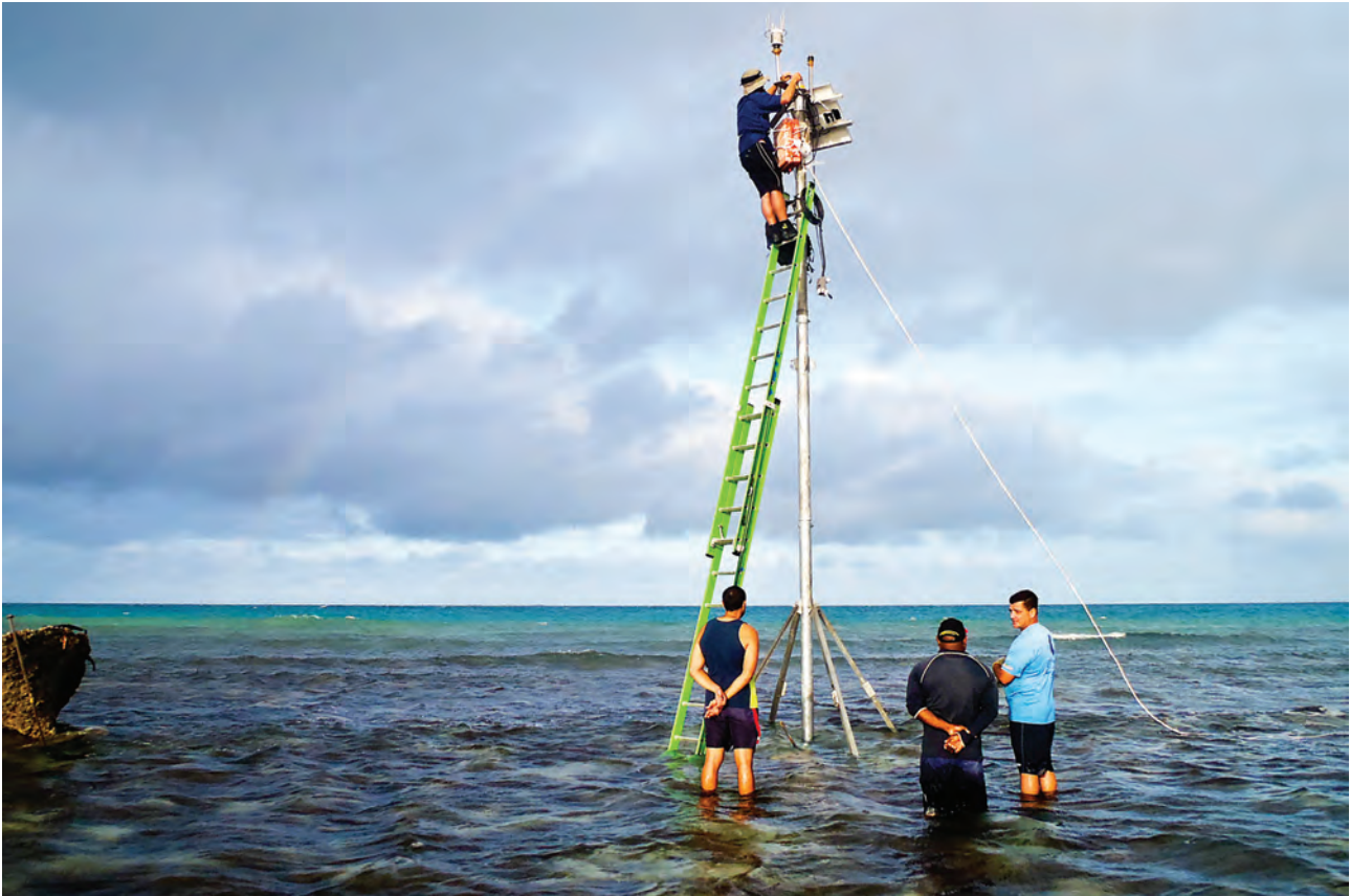
The installation of a real-time weather and ocean observing station at Masig in July 2013 will help deliver improved bleaching forecasts for the Torres Strait in summer as well as help locals with local weather data to make boating safer. Image: Scott Bainbridge (AIMS, Townsville)
